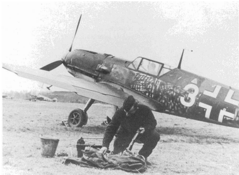
The order to darken the sides of the Messerschmitts was interpreted differently by the units. The ground crew of this 4th Staffel Bf 109E-4 took the easy route, and smeared on some RLM 02 gray paint with a brush – Marquise, Autumn 1940. ( Dölling via Petrick )
